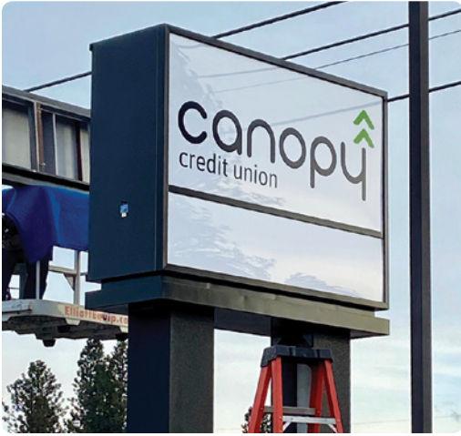
new signage going up at 1212 W. Francis
